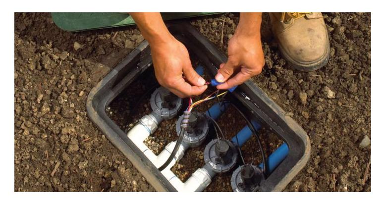
The Irritrol® 2400 Series globe and 2600 Series angle valves are popular with users because of the convenience of their threaded bonnets, the reliability of their double-beaded diaphragm and the durability of their heavy-duty, corrosion- and UV-resistant PVC construction. Fast and easy to install and service, these 1-inch residential plastic valves offer an encapsulated solenoid, internal/external bleed, an optional flow control feature, and are available in multiple configurations.
